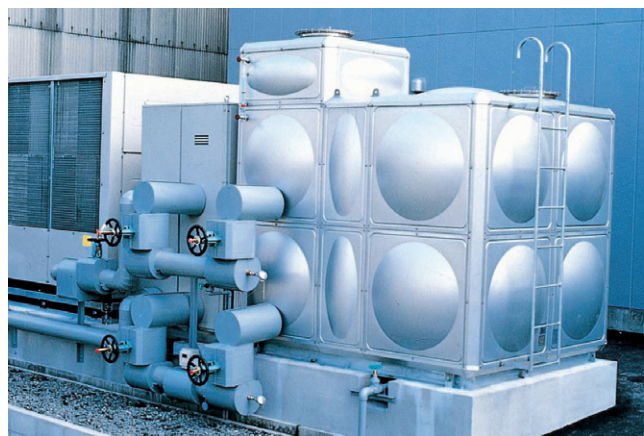
潜熱利用蓄熱槽 Heat-Storage Tank Utilizing Latent Heat
